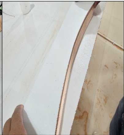
place the template and marking of arc
