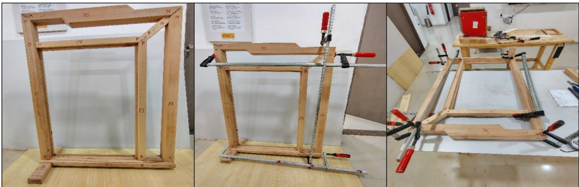
Apply glue in all joints
